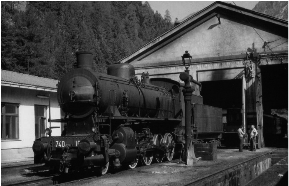
Fig. 1 – Warehouse for the locomotives, Fortezza 1975
