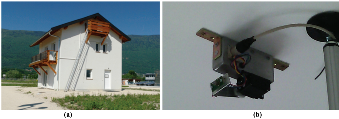
Fig. 6. (a) Building in the INES platform for the test conducted; (b) Thermal comfort system placed on the ceiling of Test Room for the test
