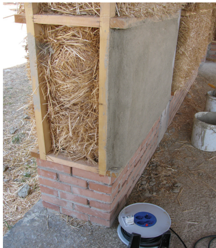
Fig. 1. Straw and raw earth plaster applied on a straw bale wall
