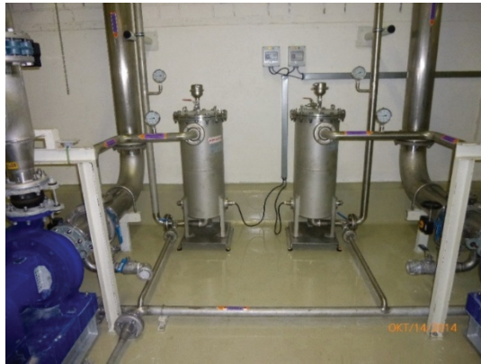
Fig. 7. MOLLIK-Module with stainless steel vessel
