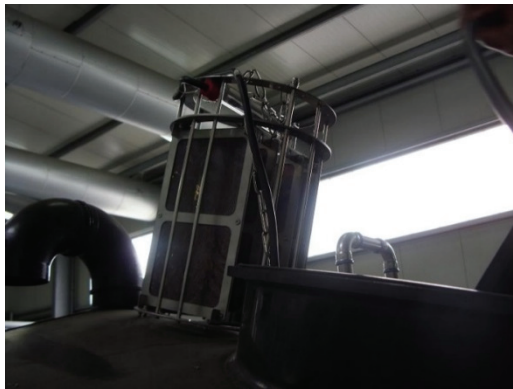
Fig. 8. MOLLIK-module during installation at feed water tank of RO
